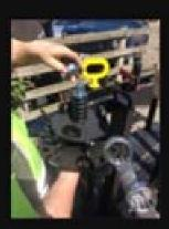
The barb spider should be placed on top followed by a washer, then the spring, washer, and nut.
