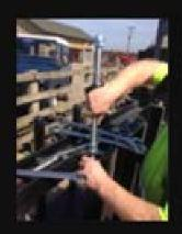
The spring bolt should now be fixed to the underside of the barb spider as shown. The barb spider should just be able to be turned by hand. Now, affix the wire support rod using the supplied nuts and washers.
